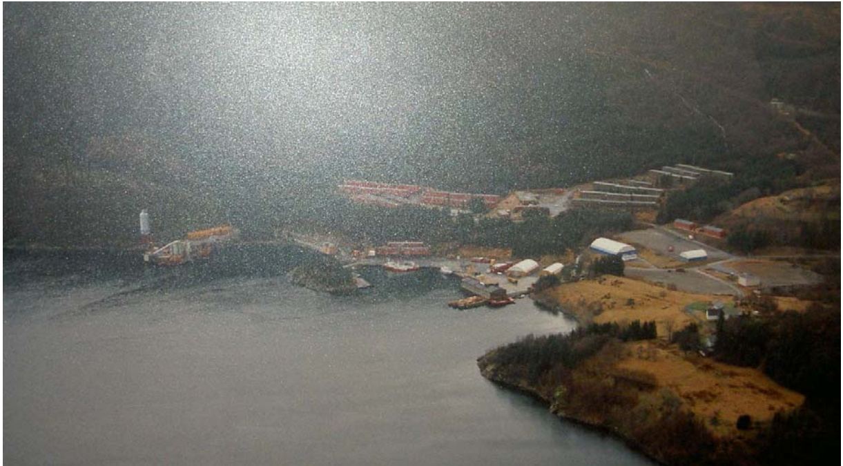
Figure A6: Overview of Raunes ca. 1991. The cement silo situated at Grønnavikskai is visible on the left hand side of the picture. Photo: Odd Furenes.
